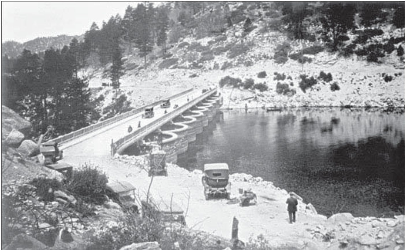
1925 Big Bear Lake; The Eastwood Dam with newly added bridge.
