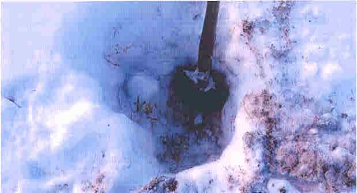
Photo 2. Hole dug to soil level along sea wall alignment in December.
